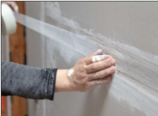
Applying drywall tape over the joints.
