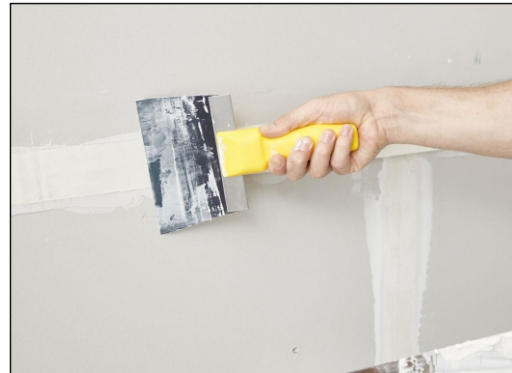
Covering the joints with a layer of jointing compound.
